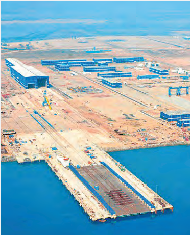
Chennai Port (L&T and Ecc Geo Structure), Tamil Nadu
