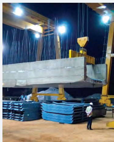
Yettinahole Aqueduct Project, Bangalore
